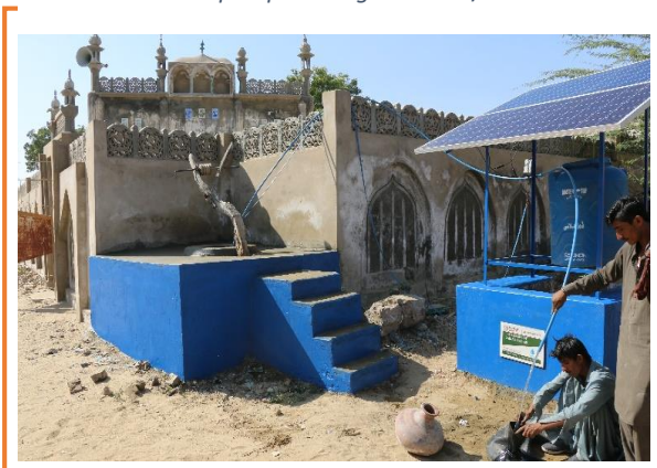
Solar submersible pump in village Dhori / Haji Sachal Muhlla
