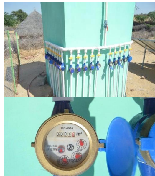
Water distribution through water meters' system in village Bhadasanda
