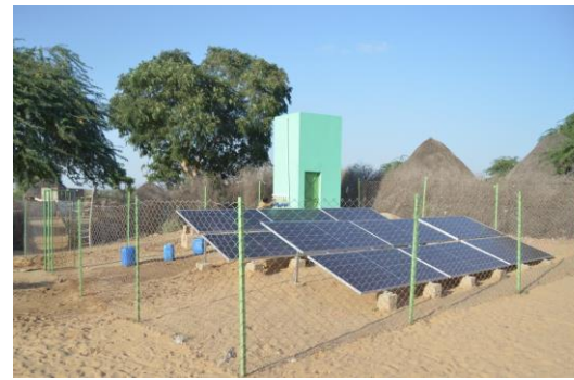
Solar powered submersible water pump in village Bhadasanda
